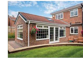
Single storey extension
