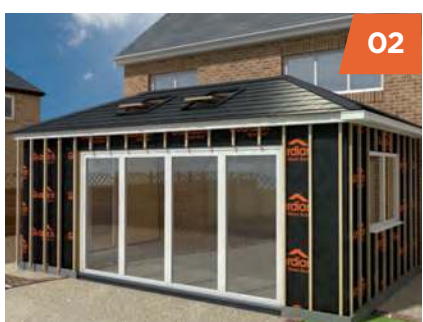
Timber battens are then secured to the outer.
