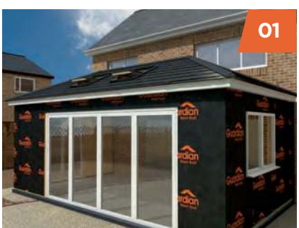
Breathable waterproof membrane is secured to the Kingspan TEK® walls.
