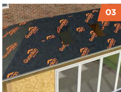
Breathable waterproof membrane is laid over the plywood and secured in place.
