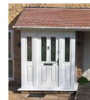
Panelled porch with decorated glass and lean-to roof.
