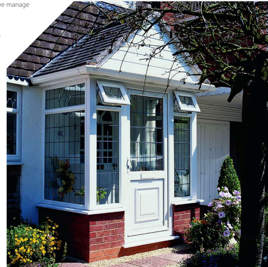
Bricked porch with clear leaded windows and gable style roof.
