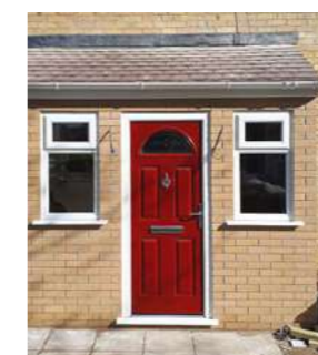
Bricked porch with clear windows and lean-to roof.
