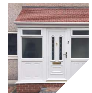
Panelled porch with obscure glass and lean-to roof.
