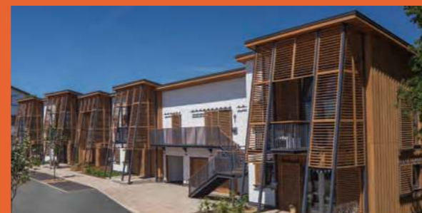
Houses, Hanham Hall, Nr Bristol Kingspan was involved from the initial design phase of the project and worked alongside HTA Design LLP.
