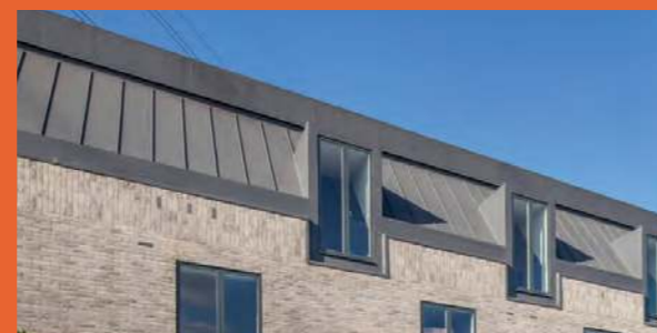
Mitcam Apartment Homes, London Built using the innovative Kingspan TEK Building System and designed by Groves Natcheva Architects.
