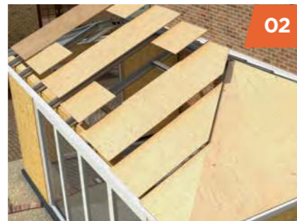
02 The aluminium roof structure is secured to the ring-beam and exterior grade ply-board is fixed.
