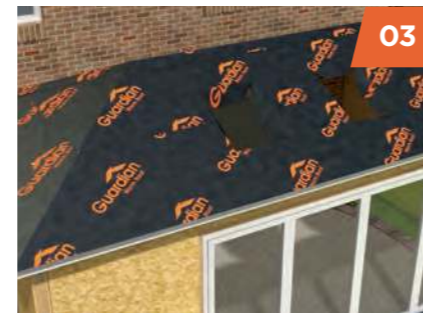
03 Breathable waterproof membrane is laid over the plywood and secured in place.
