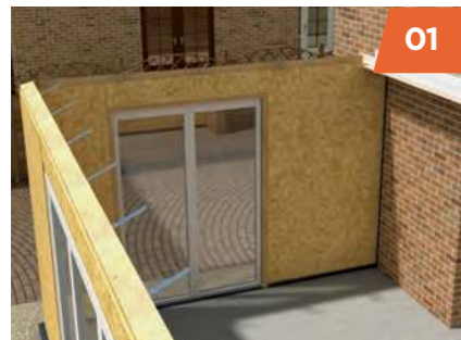
01 Structural ringbeam is sealed and secured to the top of the Kingspan TEK® wall structure.
