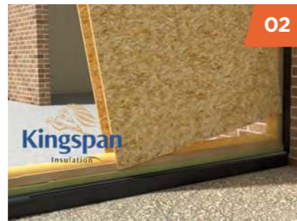
02 Wall and sole plates installed ready to receive the Kingspan TEK® panels.
