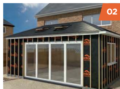
02 Timber battens are then secured to the outer.
