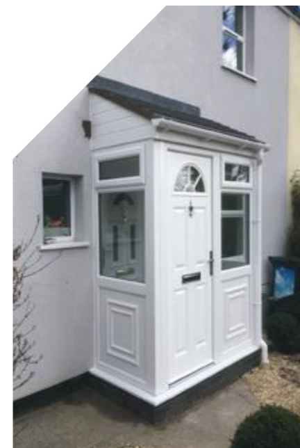
uPVC white composite door, panel sides with clear glass and lean-to tiled roof.
